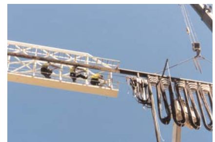
Installation on a container crane
