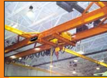
6 ton underhung double girder bridge crane with 3 endtrucks. Plastic injection molding
