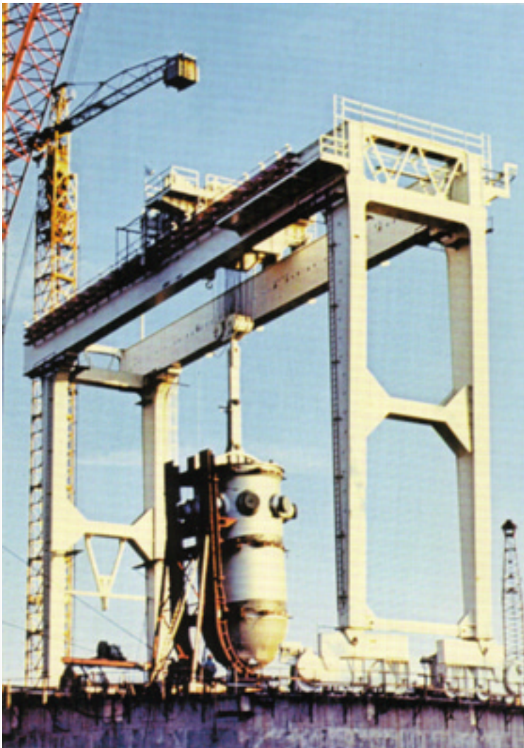
Radio controlled 460 ton polar gantry crane for reactor containment service.
