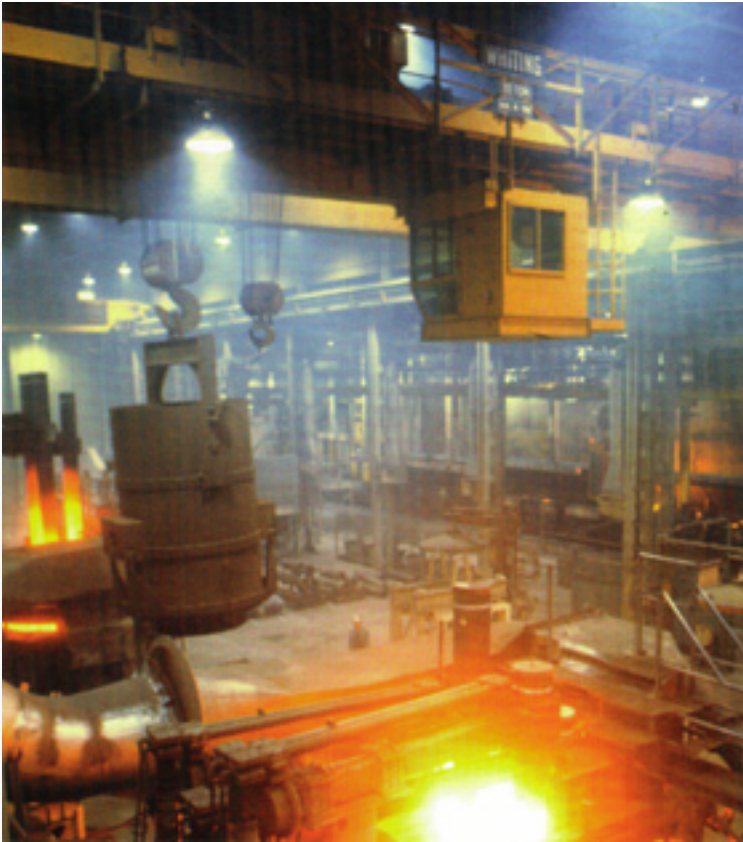
30/10 ton, center mounted cab crane working in a complete Whiting designed and fabricated equipment melt shop of a major farm equipment manufacturer.
