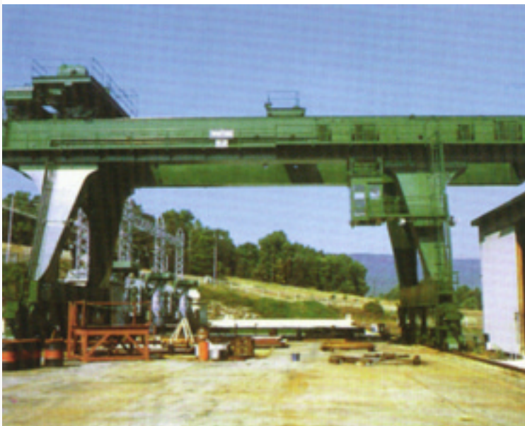
This 317 ton gantry crane performs material handling tasks at a pumped storage power generation station.
