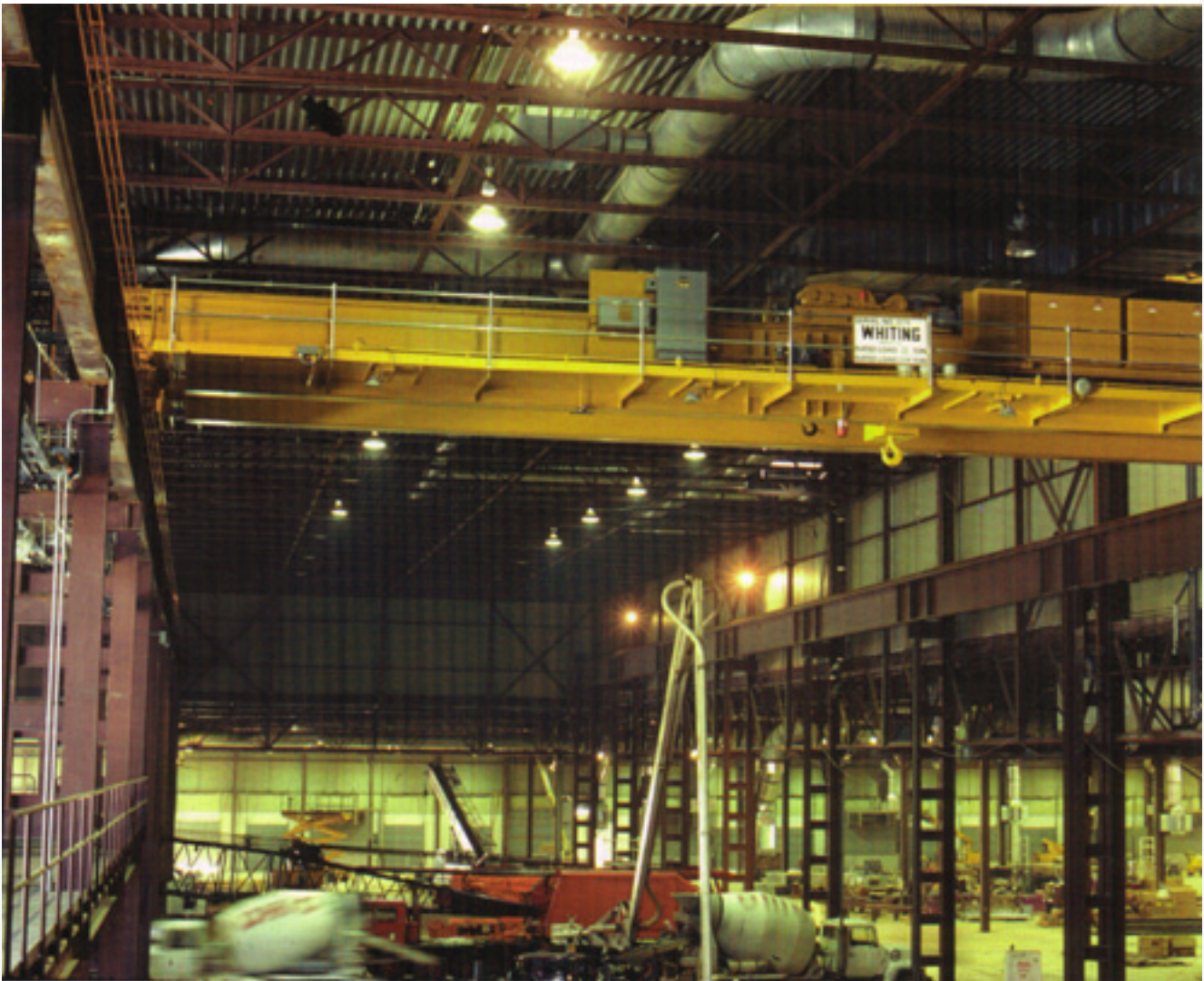
22 ton crane with a 9 ton auxiliary hoist, at work in an automotive stamping facility.
