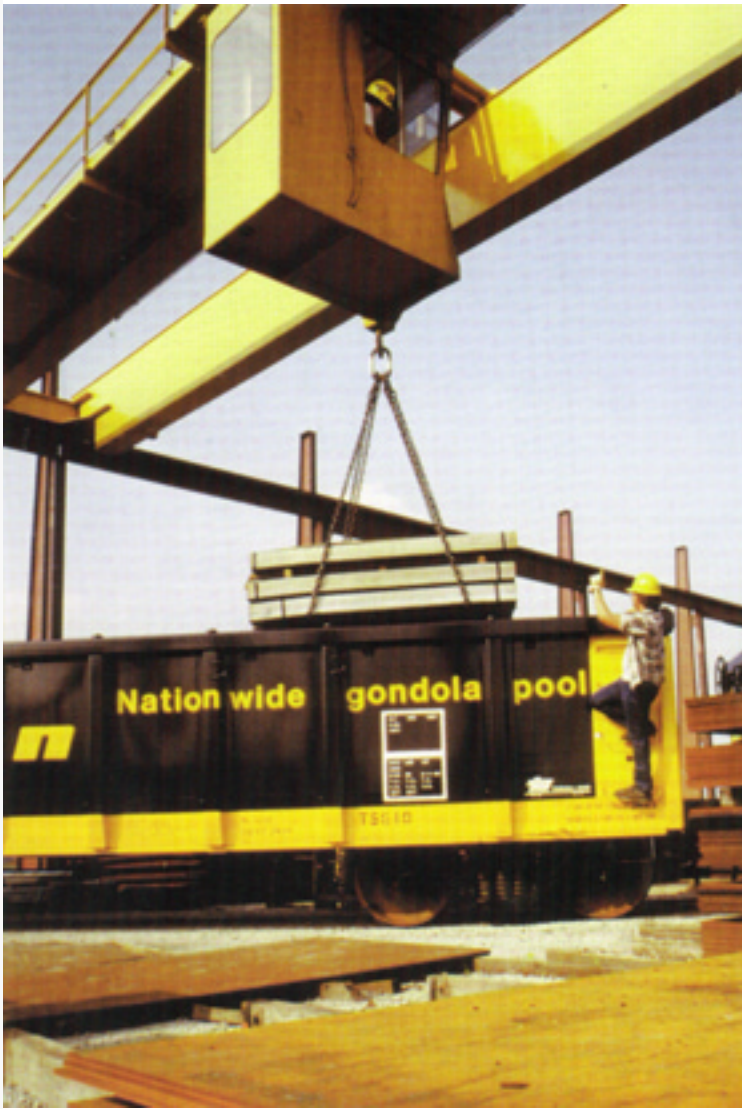
This 15 ton crane is used for moving steel In the storage yard of a major rail car manufacturer.
