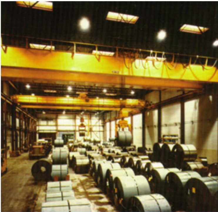
Twin, 30 ton, single trolley cranes smoothly perform coil handling tasks.
