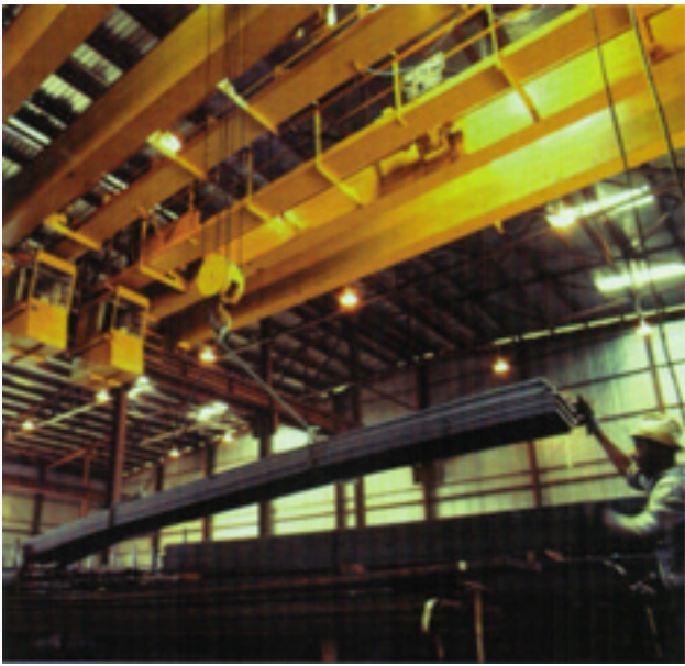
20 ton crane moving material in a steel service center.
