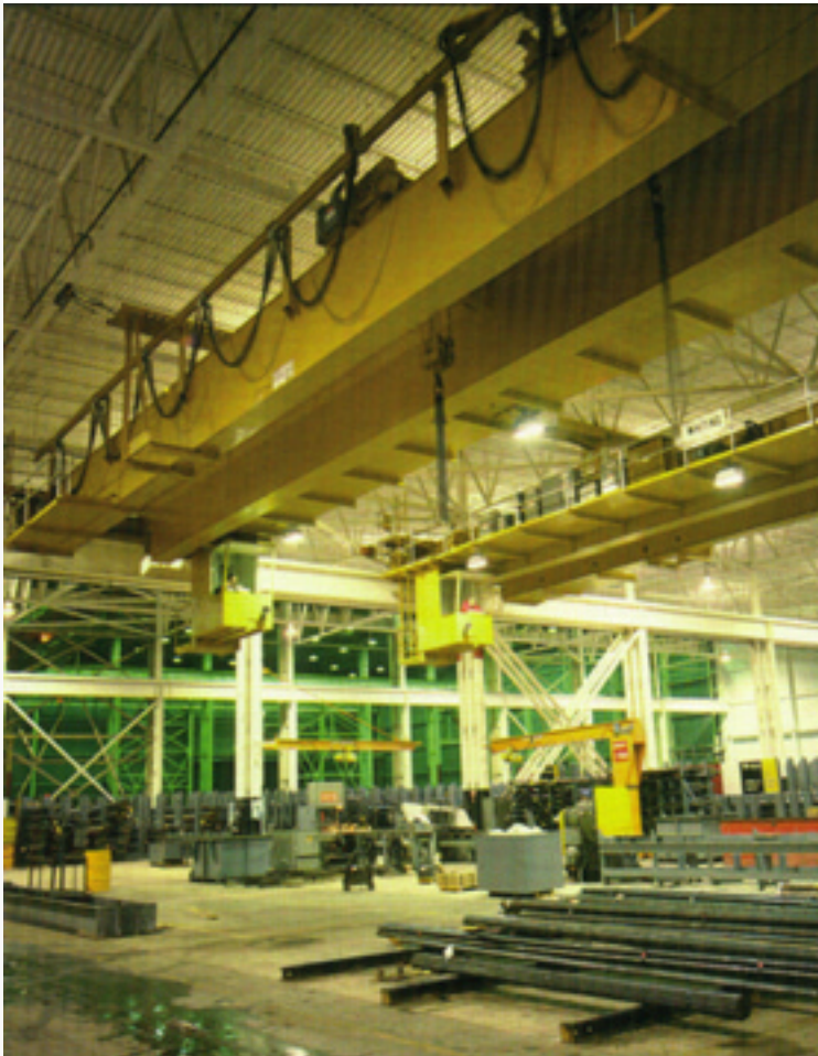
Versatile, cab controlled crane does a variety of steel warehouse handling jobs in a major mid-west steel service center.
