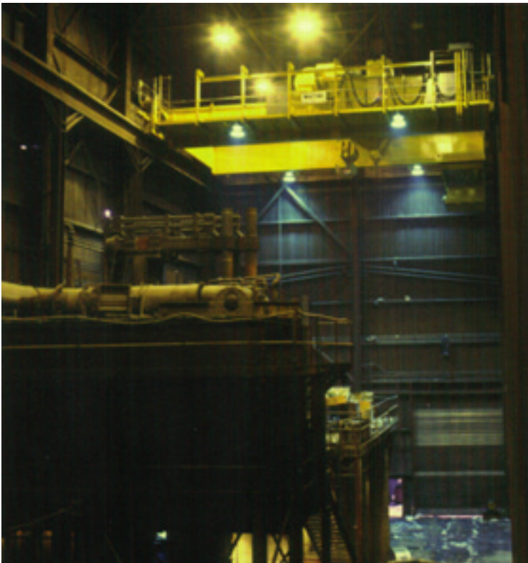
A Whiting 150/50 ton charging and hot metal handling crane services a 15'-0" diameter Whiting Hydro-Arc® Furnace.
